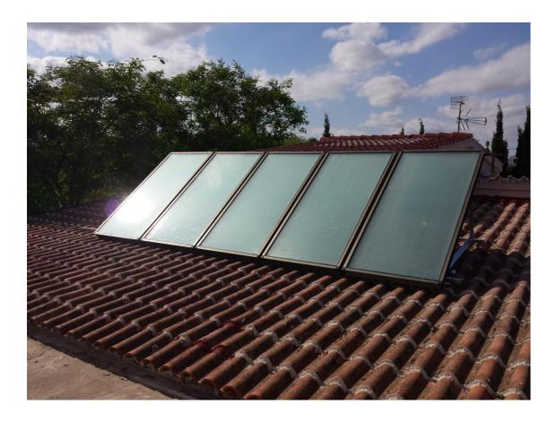
These systems have a proven track record for durability and performance and with a simple periodic safety valve check, system flush and propylene recharge every 2 to 3 years, will function at 100% efficiency and extend your yearly pool usage time for many years to come.
